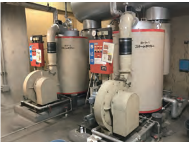
Fossil fuel boiler before decommissioning (JVCKENWOOD Nagano Corporation)
