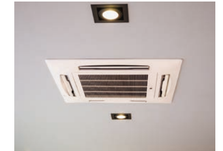
Upgrading production/air-conditioning equipment to high-efficiency models
