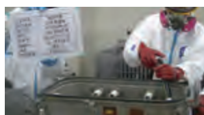
Workers extract oil at the storage facility for low density PCB contamination
