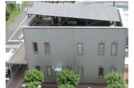
Installation of energy-saving equipment (solar power generation)
