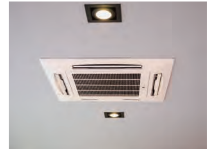
Upgrading production/air-conditioning equipment to high-efficiency models
