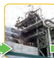
Facilities for removing insulation oil that contains traces of PCB
