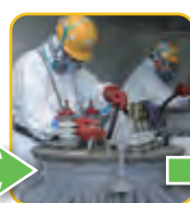
Removing insulation oil that contains traces of PCB
