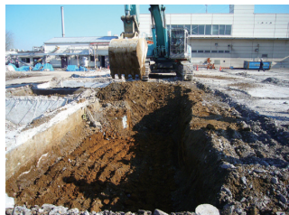
Polluted Soil Excavation Work
