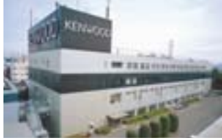
Head Office / Hachioji Business Center
